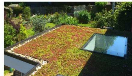
7 Example of a green roof system
