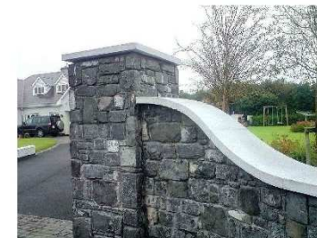
GRANITE STONE WALLS.
