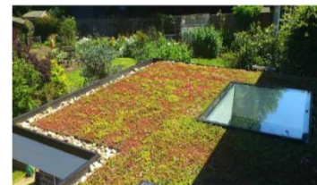
7 Example of a green roof system
