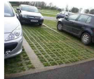
Typical Precast Concrete Paving Layout
