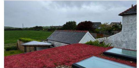
View: North West
