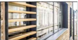
Example of: Timber Bris Soleil (Photograph indicative) Actual colour and fitting to be confirmed. Timber Bris soleil to be installed to south facing classroom windows with horizontal profile and PPC support frame.
